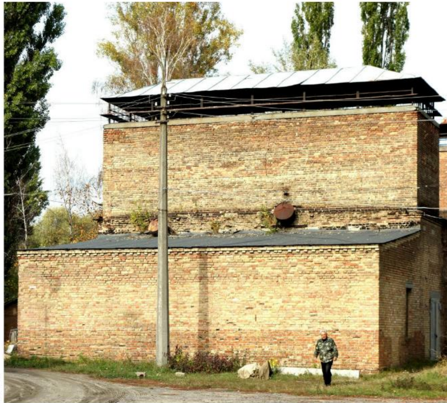
Storage and restoration area Air force museum
